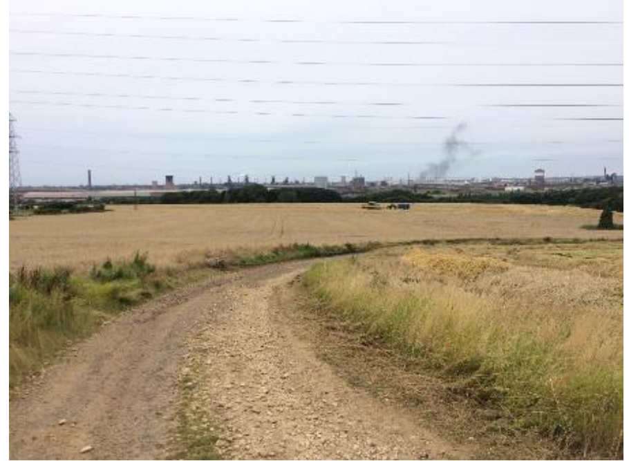
Plate 5 View west from rising ground looking towards the steel works (Figure 11, D)
