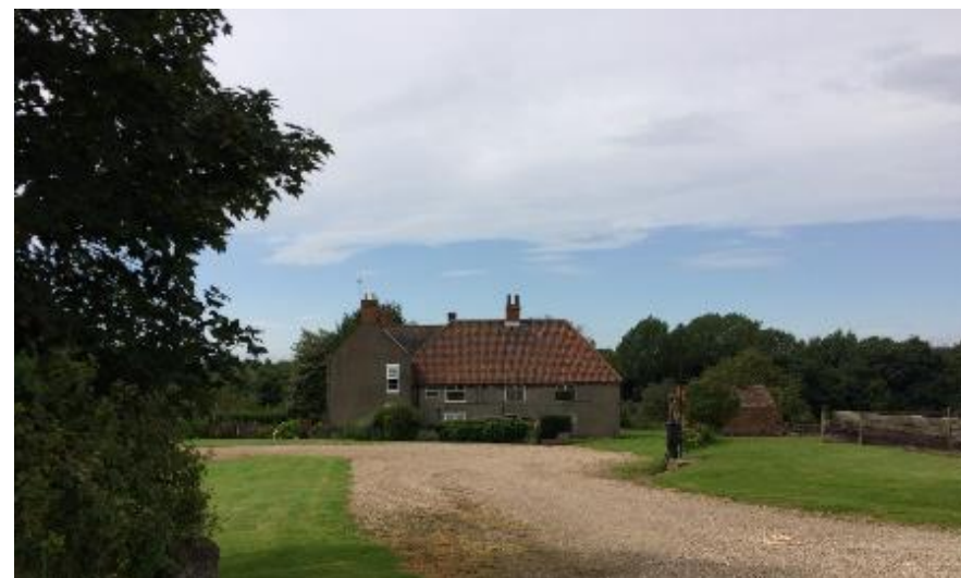
Plate 40 View west looking at Grade II Listed Raventhorpe Farmhouse
