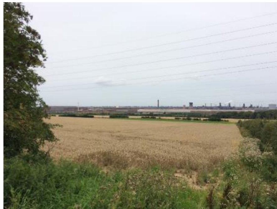
Plate 13 View southwest across the Site looking at the steel works (Figure 11, L)
